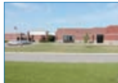
Ellsworth County Medical Center 1604 Aylward Street Ellsworth, KS 67439 Roger Pearson 785.472.3111
