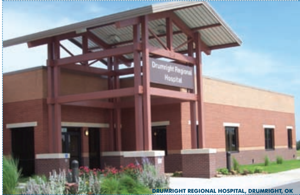
DRUMRIGHT REGIONAL HOSPITAL, DRUMRIGHT, OK
